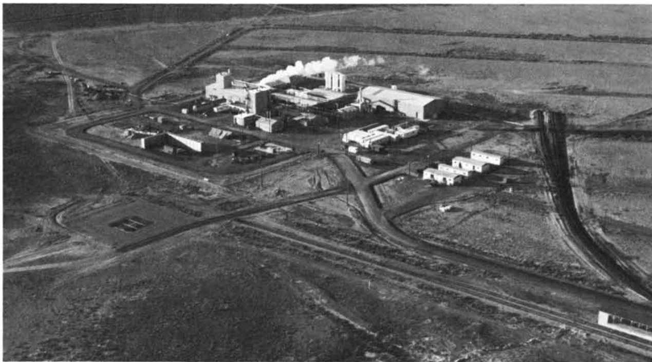
DISPOSAL FACILITY for the destruction of chemical weapons that have become unserviceable was built recently at the Tooele Army Depot. Agent GB is decomposed here by hydrolysis in alkaline solution, agent VX is decomposed by chlorination and mustard gas is destroyed by incineration. The disposal of unserviceable stocks of
